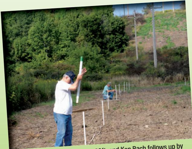
Chuck Stone drives posts every 30ft. and Ken Bach follows up by applying the 6ft. fiberglass rods and wire clips to each post. This Dr. Deer Electric Fence System took less than five hours to install over the 3-acre food plot that our "Wounded Warrior" friends will hunt on.
